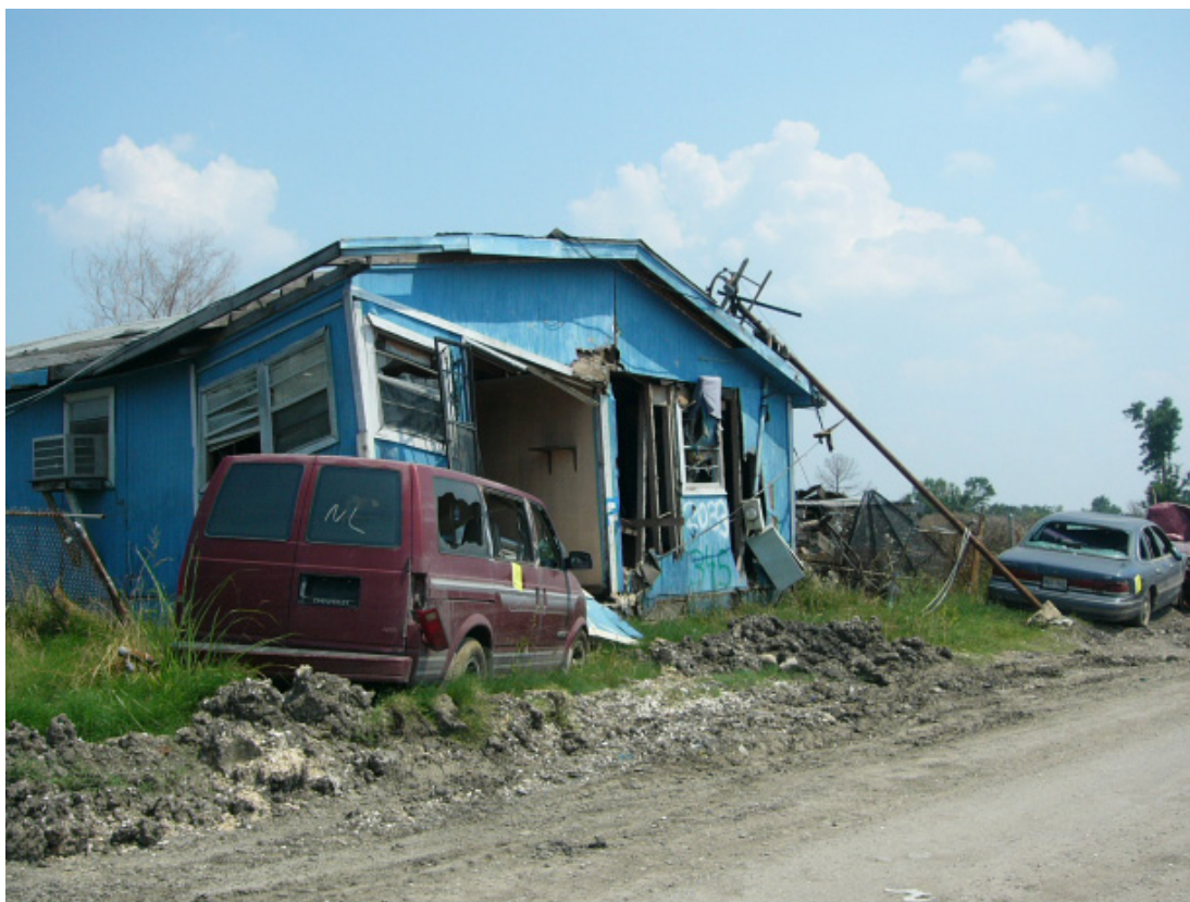
New Orleans 9th Ward, days after the floodwaters have receded, in a scene from Trouble the Water. Courtesy Elsewhere Films.
